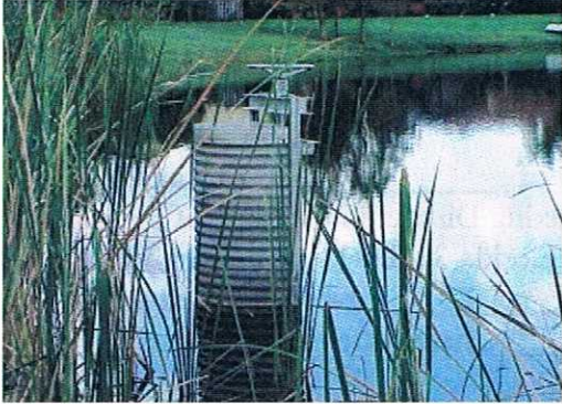
Figure 4: Example water grasses obstructing flow in Operable DCS
